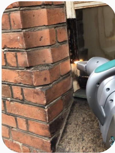
Wooden window frame of a protected building before (left) and during laser cleaning (right)
